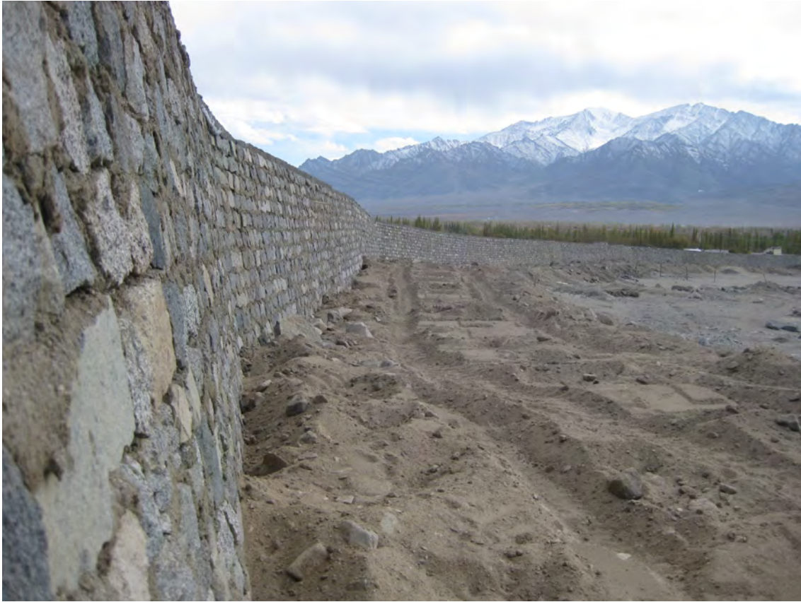
Druk White Lotus School is now protected from future mudslides by a 3m defence wall.
