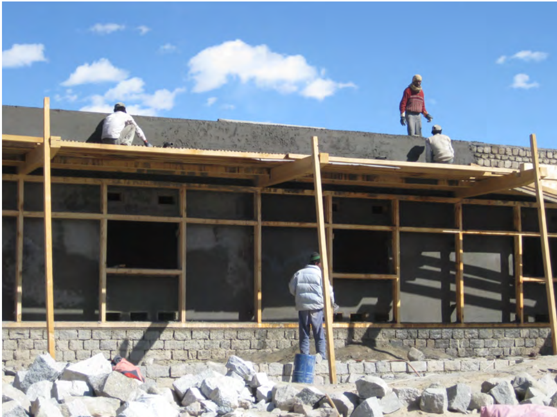
Residence 4: Rendering placed on trombe walls; roofing work almost complete.
