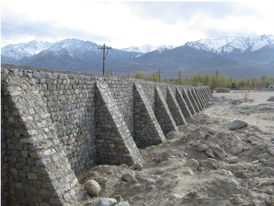
The buttressed section of the defence wall towards the southern end of the campus boundary.
