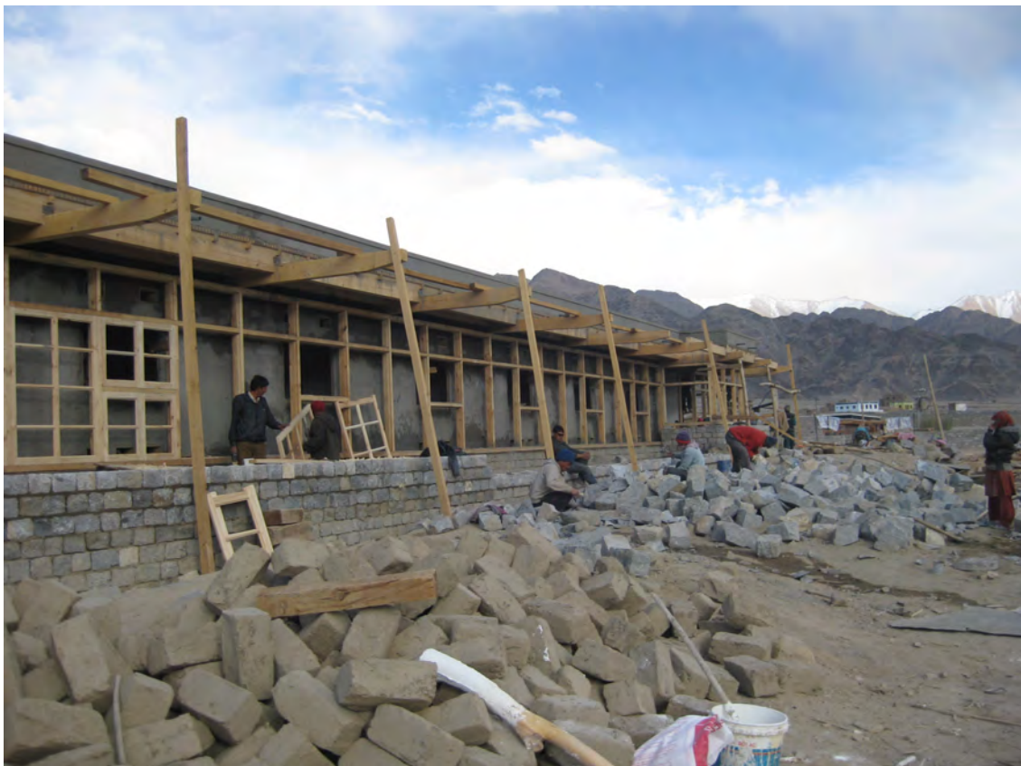
Carpenters installing the window frames in front of the Residence 4 trombe walls.
